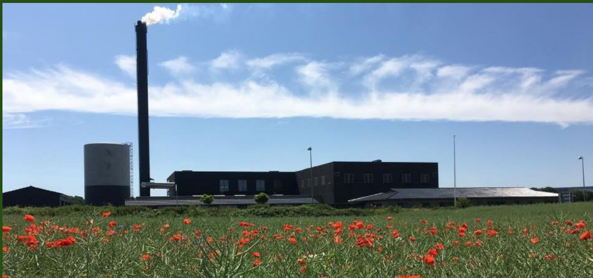
Figure 1. Heating plant in Denmark, where the willow wood chips are burned for heat production.
